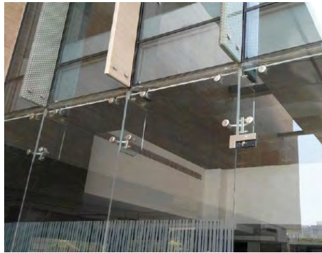
Ambience Tower, Gurgaon
